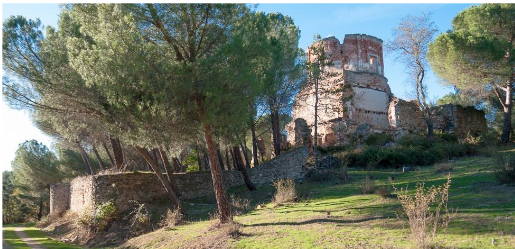
1. Forest House. General view from the S.E
