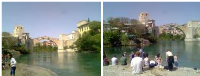
Figure 36. Old bridge in Mostar (43°20'14.16"N, 17°48'54.04"E) Source: (5.1.2013.)
